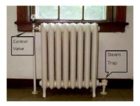
If the radiator is installed in an enclosure the capillary tube model must be used.
